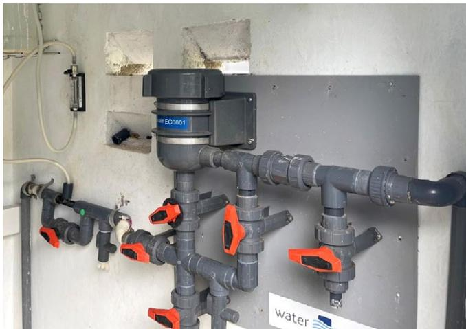
Pump Controller (left) and Erosion Chlorinator (right)
