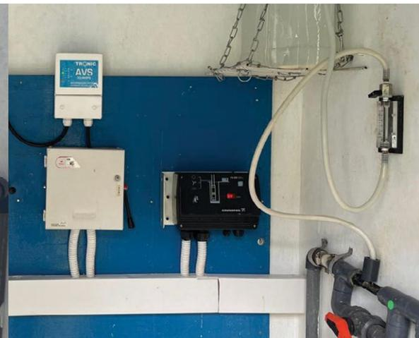
2-way Disconnect (left) and Pump Controller
