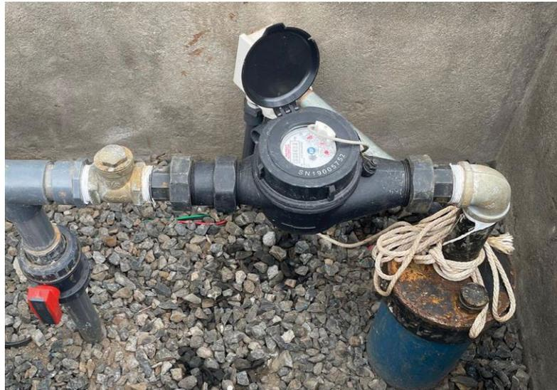
Wellhead (inside borehole cover) with piping and safety rope for submersible pump, water meter, and accessories for water level sensor.
