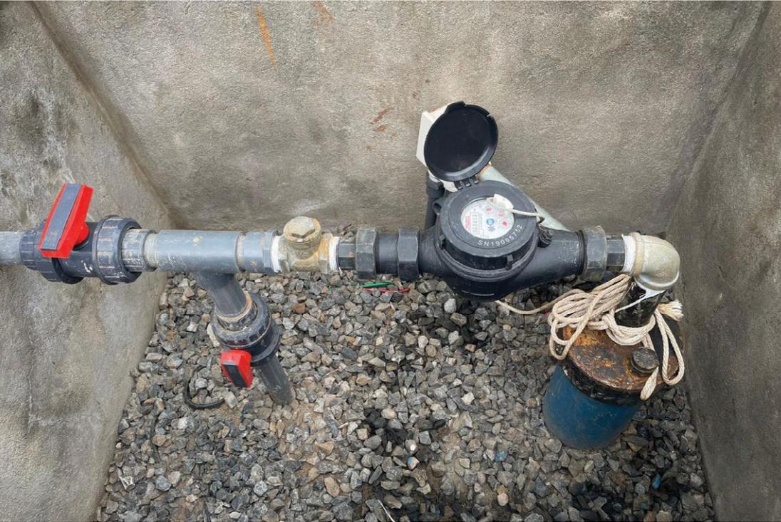
**Wellhead (inside borehole cover) with piping for submersible pump and water meter
