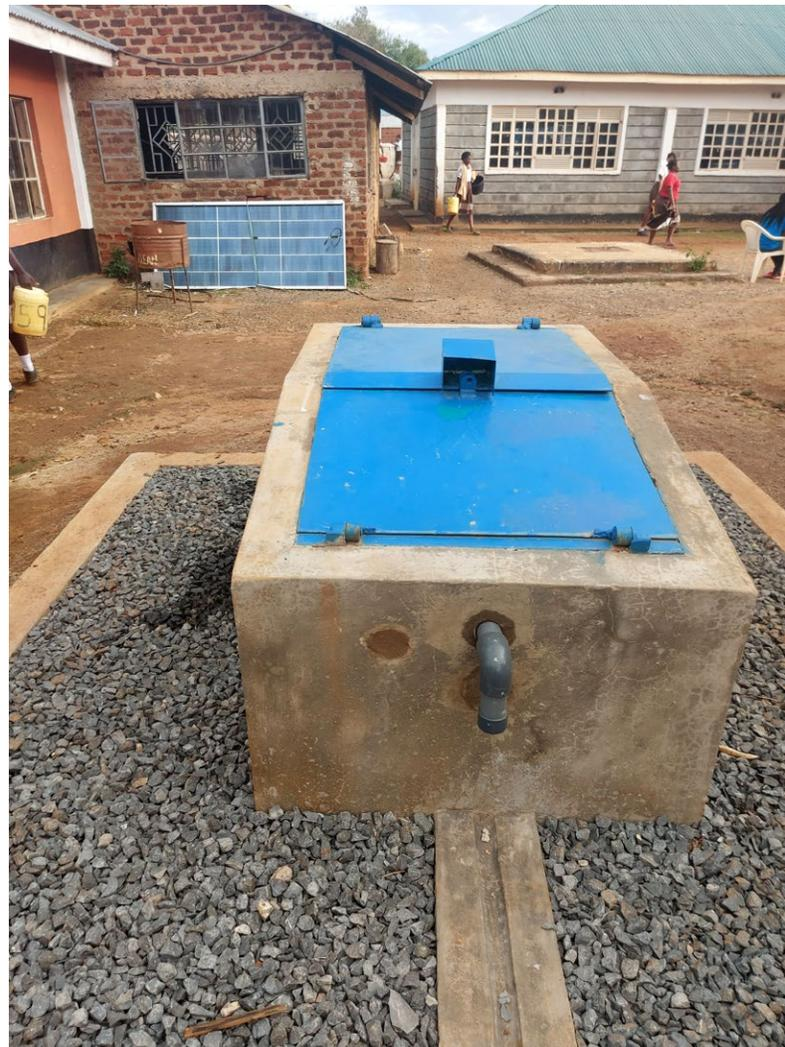
Wellhead with borehole cover at Newa Community Project (Kenya). Inside is the well with submersible pump, accessories, and piping.
